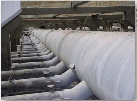
The minimum coat thickness was 80 µm and the maximum thickness was 130 µm.
