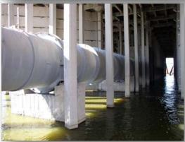
The surface preparation was done by sand-blasting followed by blowing. The Zinga coating was applied with brushes and rollers, with welding seams painted twice. ZINGA was applied in two coats.
