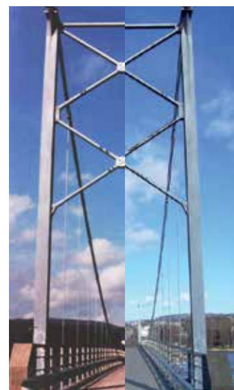
The Kalvoya bridge in Norway has been treated with ZINGA® in 1985. After 30 years, the bridge is still in good condition.
