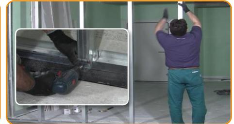
Fix the vertical metal studs on the ceiling and bottom guides by screwing
