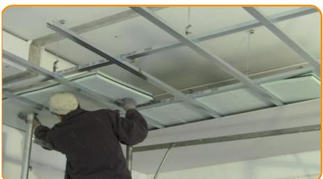
Place on top of the primary and secondary grid the insulation panels
