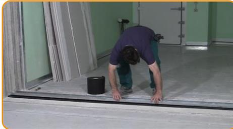
Fix metal stud on the floor, wall and ceilings
