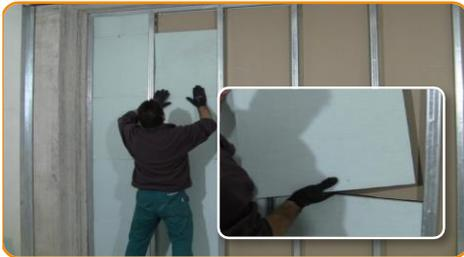
Fix the gypsum boards on one side.
