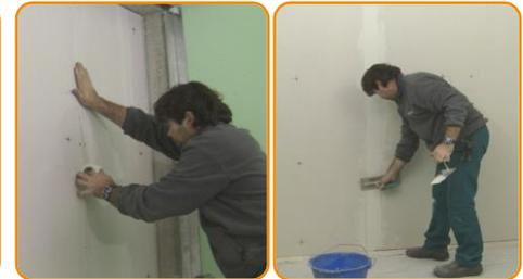
Apply the plastic mesh tape in the gypsum boards jointing lines and grouting
