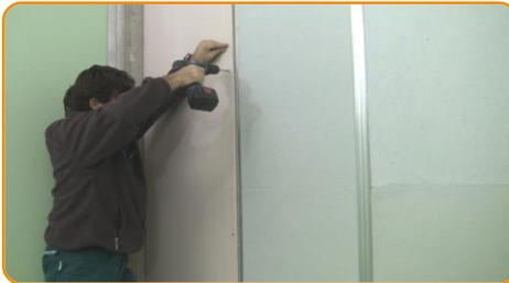
Cover the insulation layer by screwing the second gypsum boards on the metal studs
