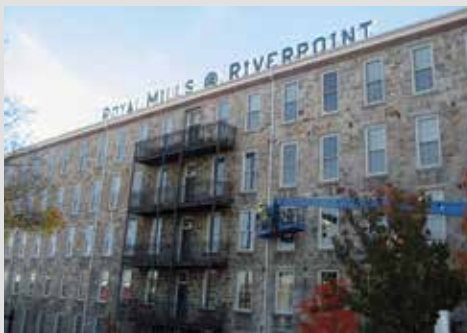
Royal Mills Riverpoint Apartments, Rhode Island, USA
