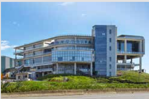
Tung Ho Steel Plant, Taiwan
