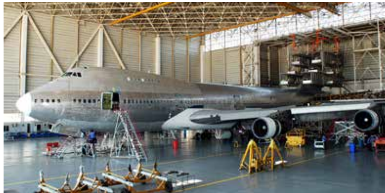
The Boeing Development Center was constructed using KIM in 1983 and has outlived its product warranty.
