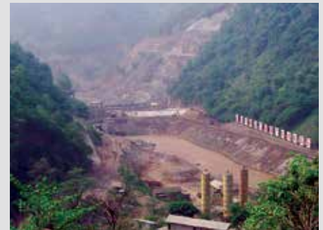
Madushan Dam, Yunnan Province, China
