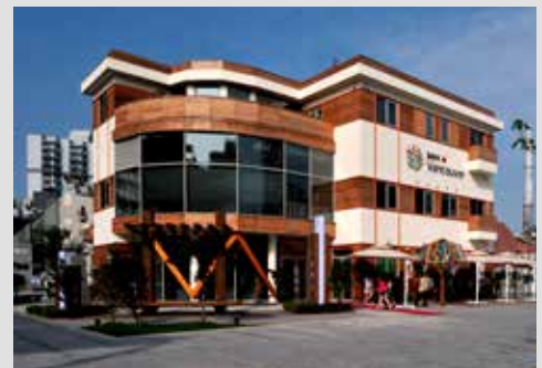
Vancouver Pavilion, Shanghai, China
