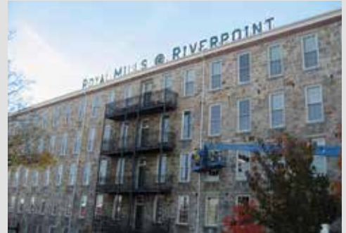
Royal Mills Riverpoint Apartments, USA
