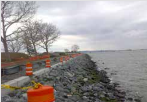
Governors Island Seawall, New York, New York
