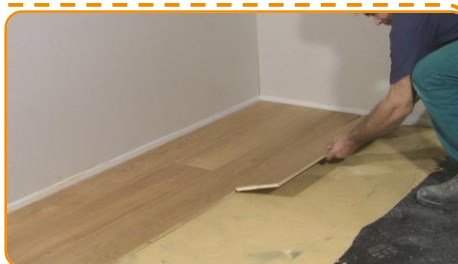
GLUE APPLICATION: apply the mat glue, then lay down the Sylwood rolls by jointing the borders with the adhesive stik tape. Glue the parquet boards over the Sylwood mat with the indicated glue.
