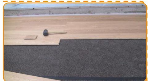
DRY APPLICATION: lay down the Sylwood and seal the roll jointing borders with the adhesive stik tape; then apply the parquet boards.
