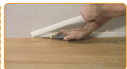
When the flooring application is completed, cut the exceeding part of the
