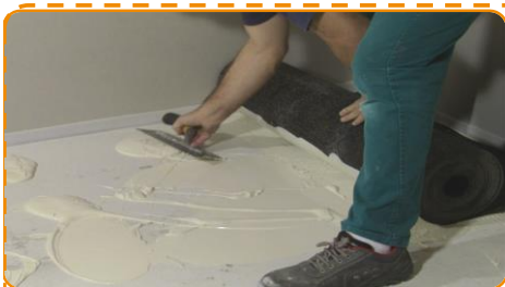
GLUE APPLICATION: apply the mat glue, then lay down the Sylwood rolls by jointing the borders with the adhesive stik tape. Glue the parquet boards over the Sylwood mat with the indicated glue.
