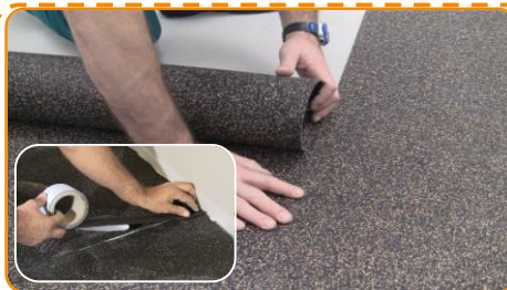
DRY APPLICATION: lay down the Sylwood and seal the roll jointing borders with the adhesive stik tape; then apply the parquet boards.
