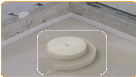
Apply the Profyle Flat 5 all along the room perimeter.
