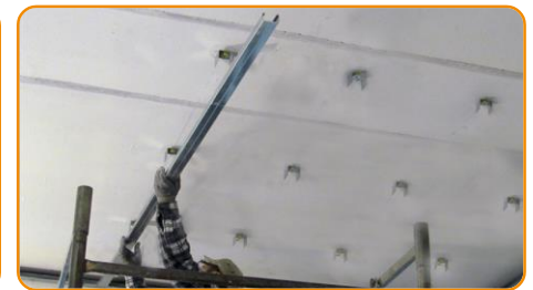
Fix the metal stud to the acoustic bracket
