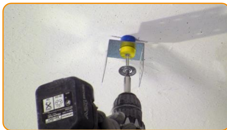
Drill the ceiling e fix the acoustic bracket
