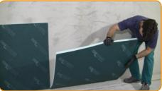
Glue the plasterboard plate to the Rewall 28R with a light pressure
