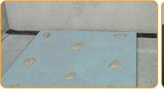
Apply the glue on the panel by spreading it on dots (suggested glue Knauf Perlfix)
