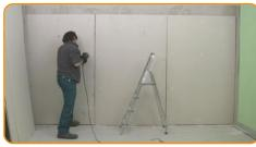
Drill the plate, the Rewall 28R and the underlying masonry as per the laying manual and fix mechanically
