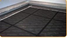
Seal the junctions between the panels with the Stik tape
