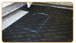
Install the edging strip to the walls and install the panels on the floor with the rubber side to the top
