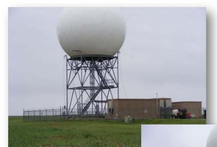
In the first half of 2009, this 10m high Nexrad tower was completely treated with ZINGA to reload the old hot-dip.
