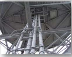
ZINGA has been applied in two coats of each 60  $\mu$ m DFT (2,5 mils) using an airless spraying gun.
