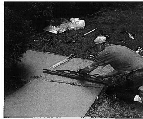
Cecil Bentley using a wooden darby to float the near the edges.
