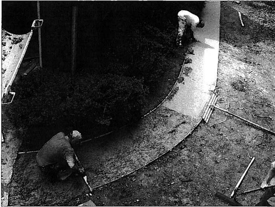
The crew struck-off, floated, and edged by hand.
