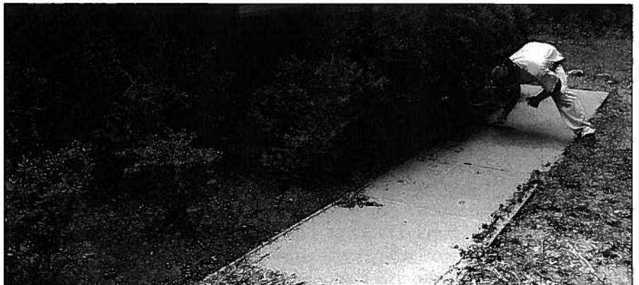
Holland and crew found placement and finishing to be no more difficult than normal, in spite of the high volume of fibers.
