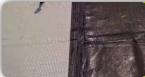
Junction between Bituver Megaver California and previous traditional membrane.
