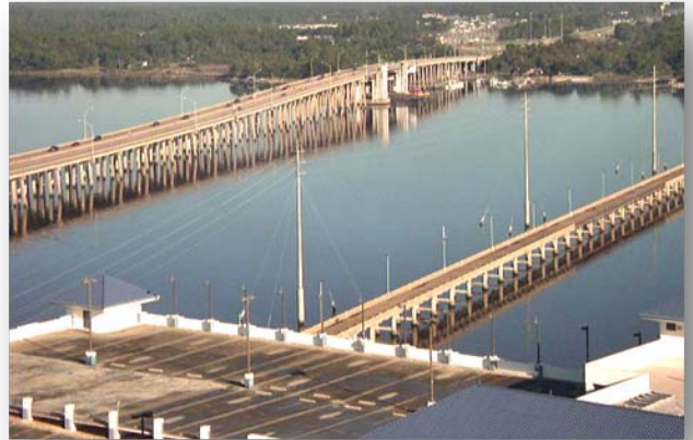
Biloxi, Back Bay Bascule Bridge (MDOT US 1-110)
