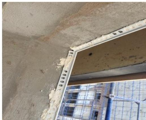
very precise. Four mixers and three pumps were used to ensure optimum mixing. Tejais reinforcing mesh was installed wherever joints are located, including stop beads at corners and abutments, and forming dip over openings. Specially-designed jointing accessories, Juntis and aluminum plasertops, were used as well.
