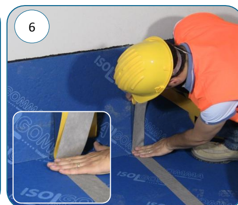
Seal the vertical joints of the mats with the Stik WP tape
