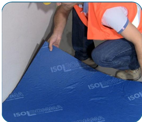
Lay the Matrack mats on the pit, without leaving gaps between adjacent mats or along the edges
