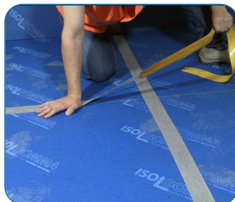
All the lines of junction have to be taped
