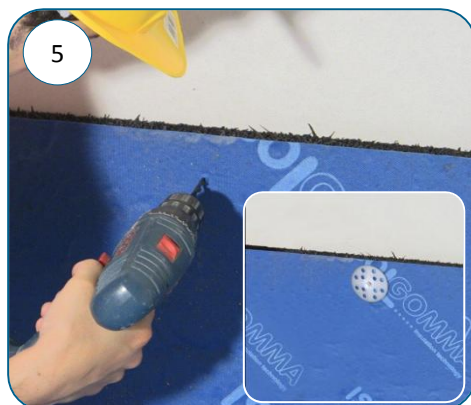
Fix the vertical mats with large headed screws or with adequate glue
