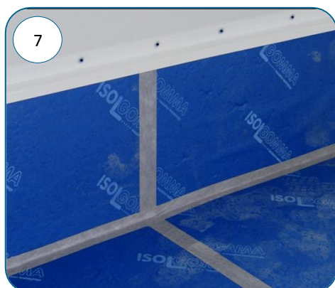
Fix the "Z" profile on the top border of the vertical mat
