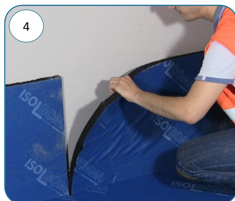
Place the Matrack mats vertically
