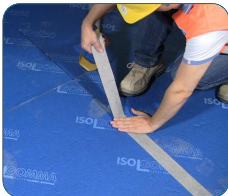
Seal the edges of the mats with Stik WP tape, taking care of the good adhesion of the tape to the mats
