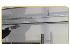
Insert the metal stud of secondary grid in the perimeter channel
