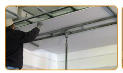
Fix the gypsum board by screwing
