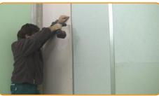
Cover the insulation layer by screwing the second gypsum boards on the metal studs
