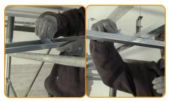
Fix the metal stud of secondary grid to the primary grid with the appropriate connector
