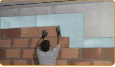
Apply in the first wall a layer of row mortar Build the second wall with the same process of the first one and insert the panel in the
