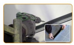
Glue the adhesive strip Stywall S3A to the metal studs and fix them along the perimeter of the room at a fixed distance from the ceiling
