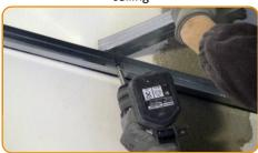
Fix the metal studs of primary grid along the perimeter channel
