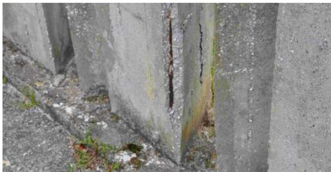
Rising-damp in reinforced concrete structures, appears usually in elements in contact with ground.
