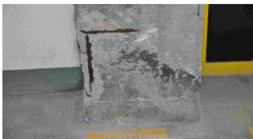
The rust cleaning on reinforcements is done by: aluminium silicate blasting, needle-gun or wire brush.
