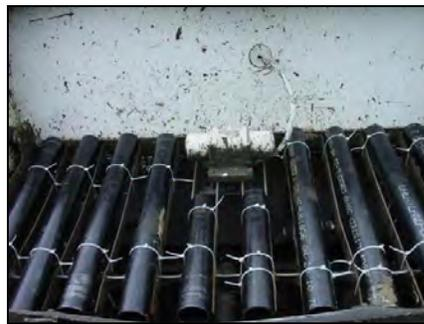
**Temporary metal pipe lay-over method zip-tied in place**
