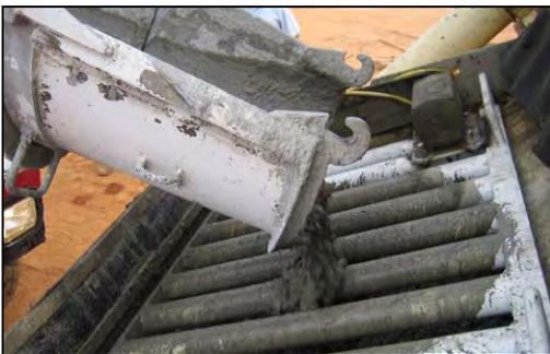
**A permanent round-bar grate is essentially self-cleansing at high fiber dosages.**
