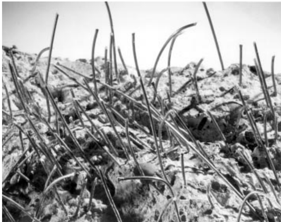
Fig. 2.1—Fracture surface of SFRC
