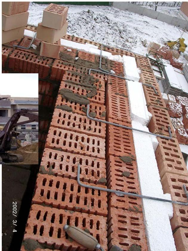
In March 2002 ZINGA was applied on rebars to reinforce the walls of a large building in Russia.
