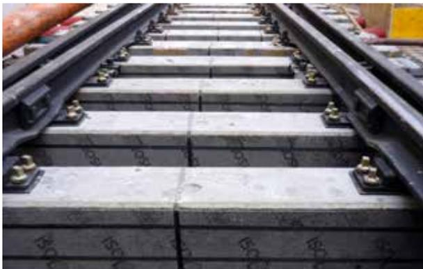
Slitrack su ballast / Slitrack on ballast
