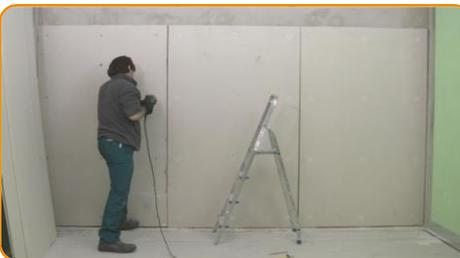
Drill the plate, the Rewall 28R and the underlying masonry as per the laying manual and fix mechanically
