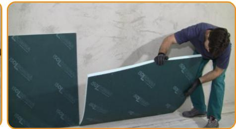
Glue the plasterboard plate to the Rewall 28R with a light pressure
