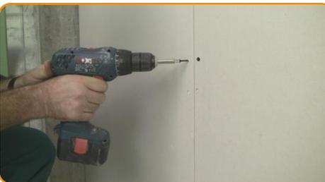
Fix the second gypsum board by gluing dots or screwing it on centre line and on the side borders with double thread screw. Offset the first board with the second
