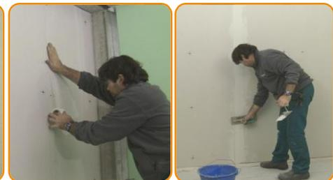
Apply the plastic mesh tape in the gypsum boards jointing lines. Grouting
