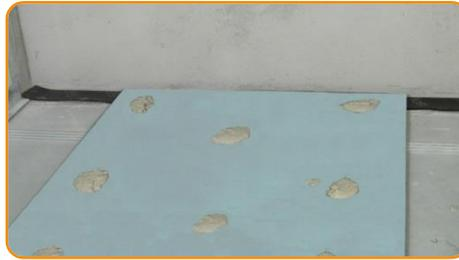
Apply the glue on the panel by spreading it on dots (suggested glue Knauf Perifix)
