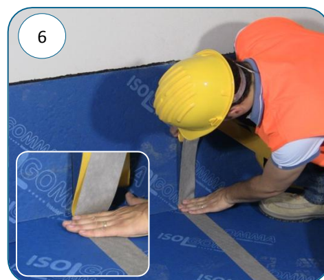
6 Seal the vertical joints of the mats with the Stik WP tape
