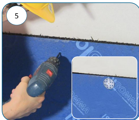
5 Fix the vertical mats with large headed screws or with adequate glue
