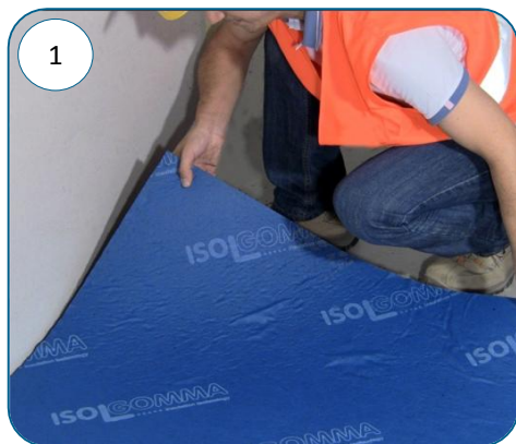
1 Lay the Matrack mats on the pit, without leaving gaps between adjacent mats or along the edges
