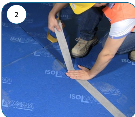
2 Seal the edges of the mats with Stik WP tape, taking care of the good adhesion of the tape to the mats
