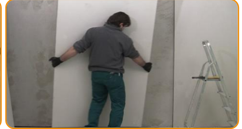
Build the screed
