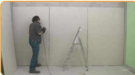
Fix the second gypsum board by gluing dots or screwing it on centre line and on the side borders with double thread screw.
