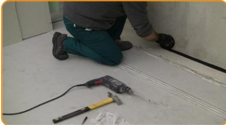
Install the edging strip to the walls and install the panels on the floor with the rubber side to the top
