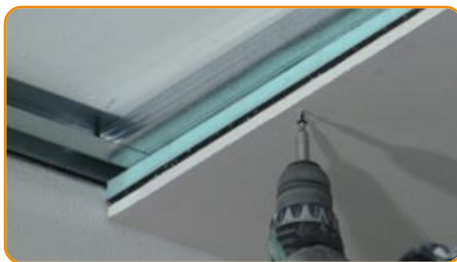
Fix the Mustwall B panel to the metal frame with 55 mm screws every 15 cm
