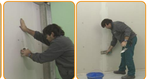
Grouting COATED CEILING
