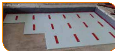
Posare i pannelli Highmat in file contigue Place the Highmat panels in adjacent rows
