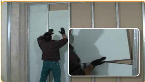
Fix the gypsum boards on one side.
