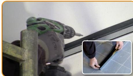
Glue the adhesive strip Stywall S3A to the metal studs and fix them along the perimeter of the room at a fixed distance from the ceiling
