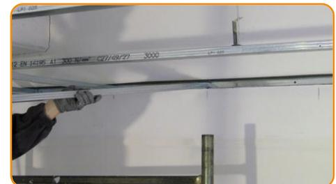
Insert the metal stud of secondary grid in the perimeter channel
