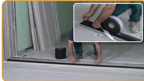
Glue on the metal studs the adhesive strip type Stywall S3-A and fix them on the floor, wall and ceilings
