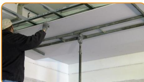
Fix the gypsum board by screwing
