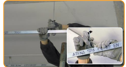
Fix to hangers the metal studs of primary grid
