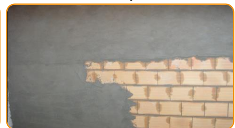
Realize the final plastering.
