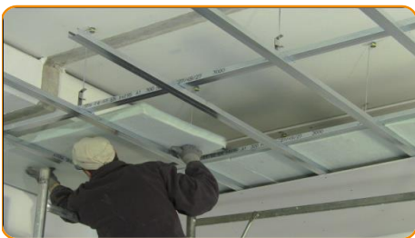
Place on top of the primary and secondary grid the insulation panels
