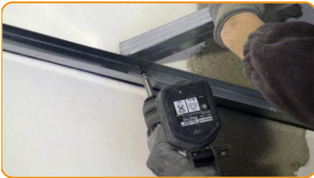
Fix the metal studs of primary grid along the perimeter channel
