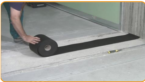
Lay the under wall strip in the dry floor.
