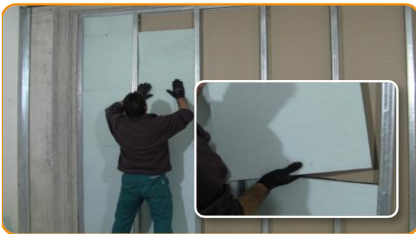
Fix the gypsum boards on one side. Insert the Fybro panel
