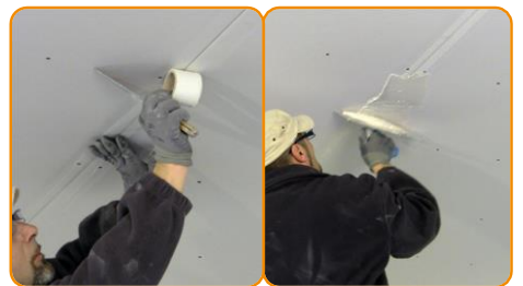
Apply the plastic mesh tape in the gypsum board jointing lines Grouting
