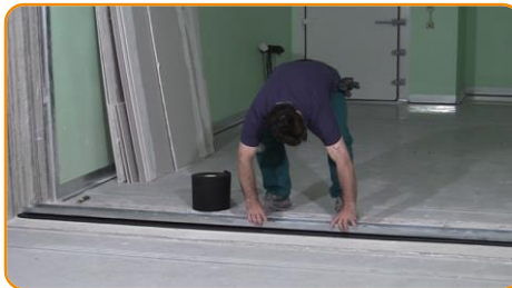
Fix metal stud on the floor, wall and ceilings
