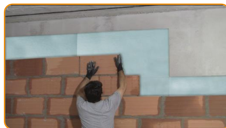
Build the second wall with the same process of the first one and insert the panel in the cavity
