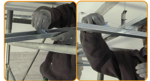
Fix the metal stud of secondary grid to the primary grid with the appropriate connector
