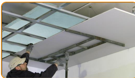
Lean the gypsum board to the metal frame Fix the gypsum board by screwing
