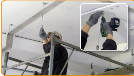
Mark and fix the acoustic hangers
