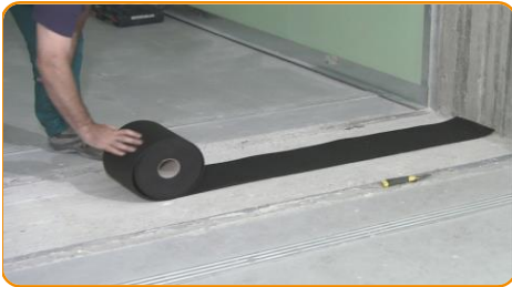
Lay the under wall strip in the dry floor.
