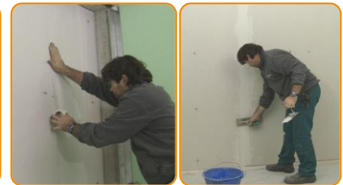
Apply the plastic mesh tape in the gypsum boards jointing lines and grouting
