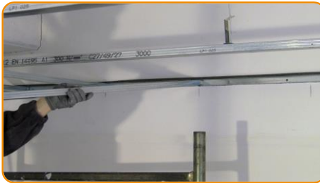
Insert the metal stud of secondary grid in the perimeter channel
