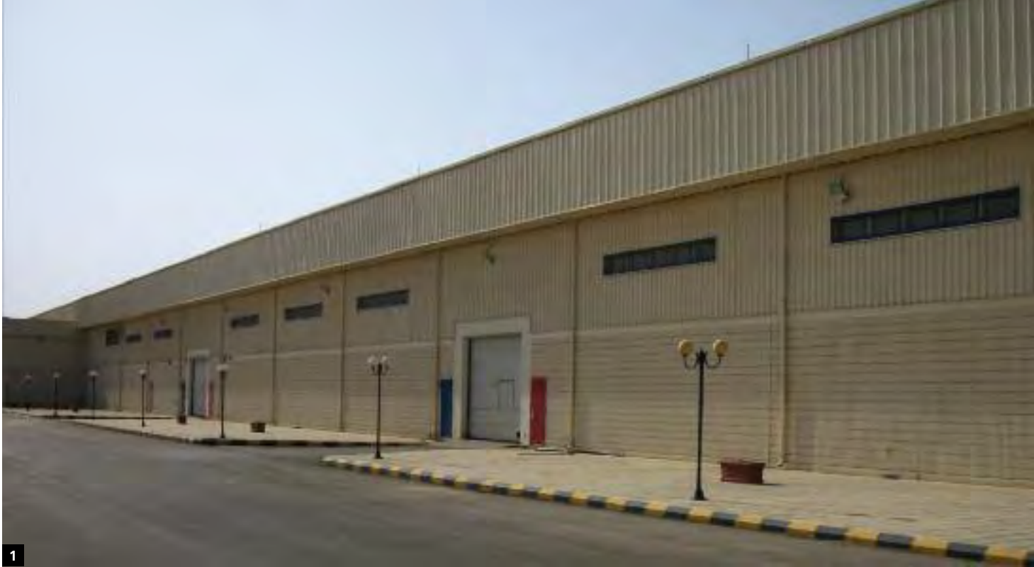
1 Industrial building, cold store.
