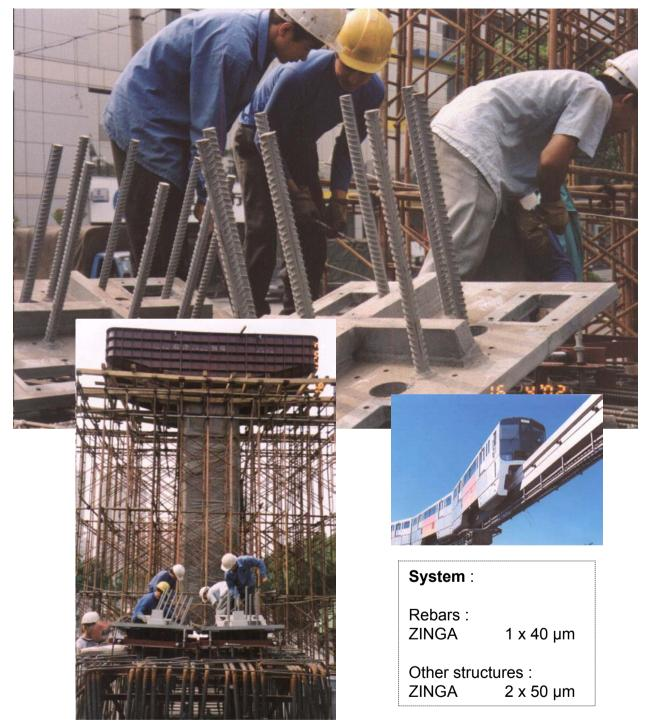
The company Chongqing Water Turbine Works (CWTW) is one of the main contractors for the construction of the Chongqing Monorail. The CWTW has applied ZINGA with satisfactory results on the rebars of the beam supports, directing splitter tracks and connecting plates. These pictures were taken on 16/04/02.
