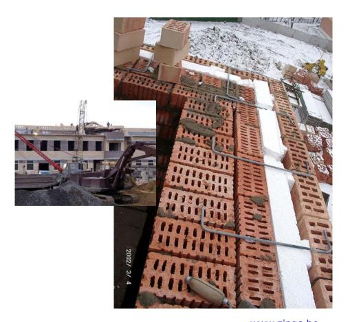
In March 2002 ZINGA was applied on rebars to reinforce the walls of a large building in Russia.
